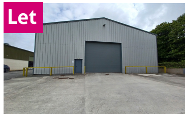
Let Modern industrial unit
