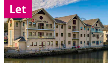
Top floor office suite
