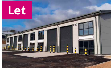
New industrial units
