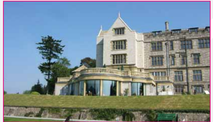
Bovey Castle – Building defect litigation
